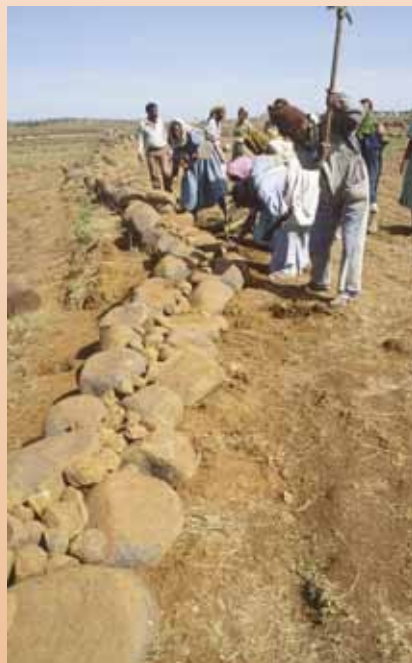
Villagers in Ethiopia using stones to create terraces, a technique to prevent soil erosion.
