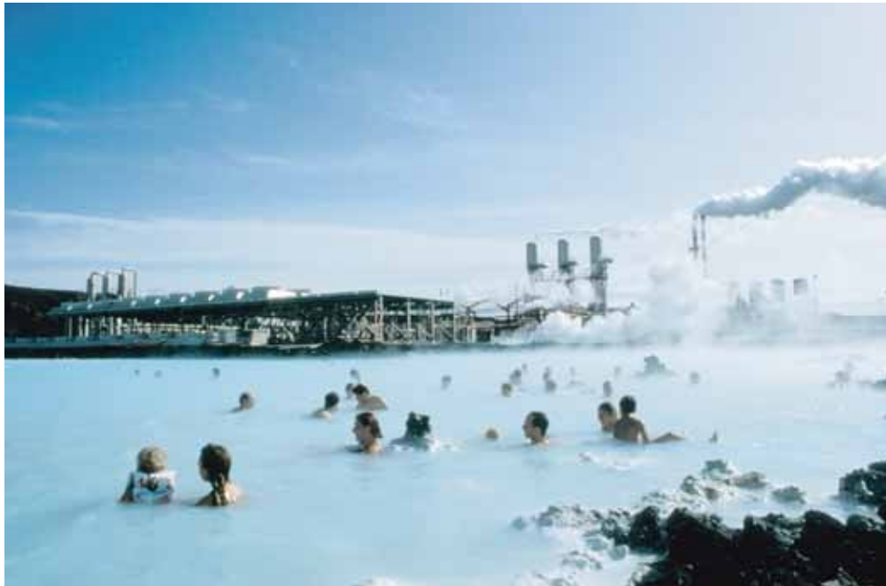
Geothermal power plant, Iceland.
